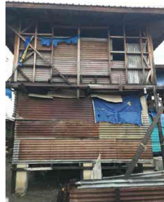
Figure 25: Incremental addition of wall finish (temporary) but structure built well. Location: Ontong Java settlement (Photo credit: John Clemo)
